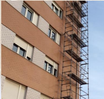
Residential Complex (Santander - Spain)
