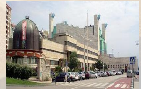
School of Marine Engineering (Santander - Spain)
