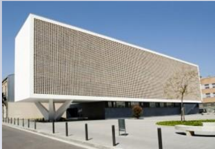
Primary Care Center- Badalona (Barcelona - Spain)
