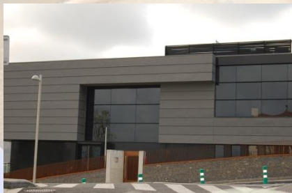
GBB Building (Guipúzcoa - Spain)
