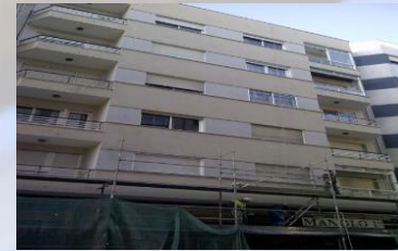
Residential Complex – Vigo (Pontevedra - Spain)
