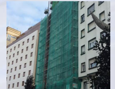
Residential Complex (Santander - Spain)
