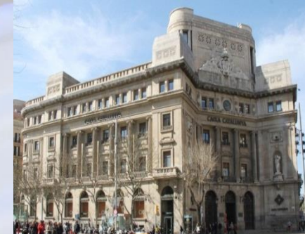
Catalunya Caixa Bank Headquarters (Barcelona - Spain)
