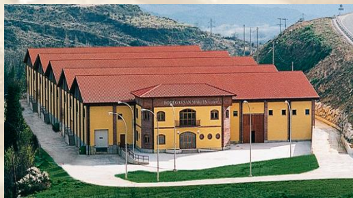
San Martin Winery – S. Martín de Unx (Navarra - Spain)
