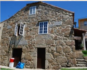
Granite Houses (Pontevedra - Spain)
