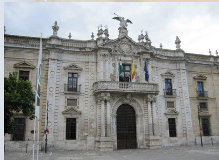
Rectorate Building – Old Tobacco Factory (Sevilla - Spain)
