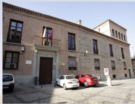
Marquis of Malpica Palace (Toledo - Spain)
