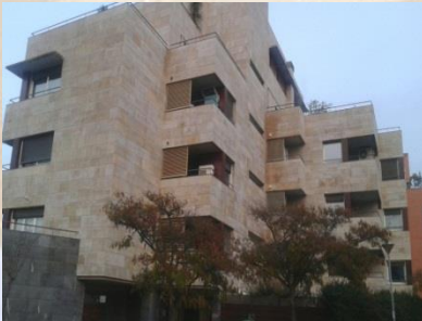
Residential Complex- Tudela (Navarra - Spain)
