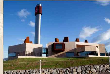
CPD Building – Santander Bank (Santander - Spain)
