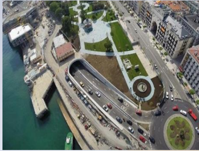
Botín Center Tunnel – Santander Bank (Santander - Spain)
