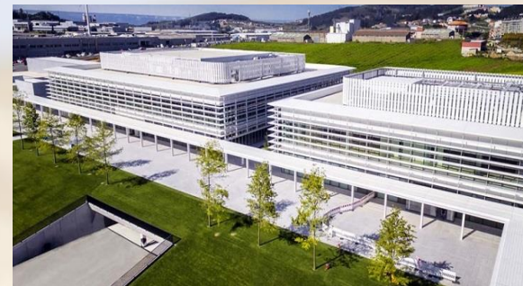
New headquarters of INDITEX – Arteixo (A Coruña - Spain)
