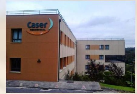
CASER Nursing Home (Bilbao - Spain)
