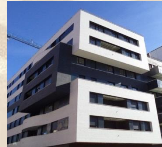
Residential Complex (Logroño - Spain)
