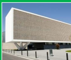
Badalona Primary Care Centre (Barcelona, Spain)
