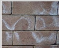
Crystallized efflorescence
