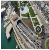
Botín Center Tunnel Santander Bank (Santander)
