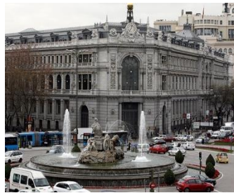
Head Office Banco de España (Madrid, Spain)
