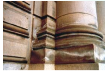
Efflorescence
