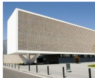
Primary Care Centre of Badalona (Barcelona, Spain)
