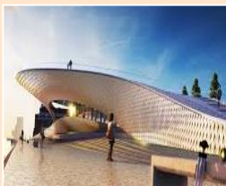
MAAT Building (Lisboa, Portugal)
