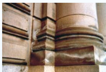
Efflorescence
