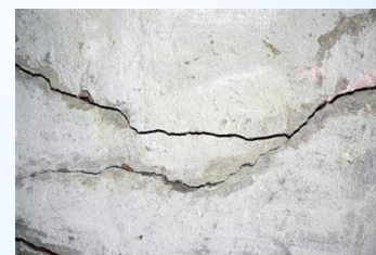
Freeze-thaw damage
